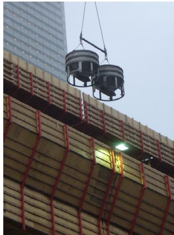
**Figure 11 – Concrete placement by bucket**
