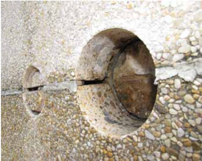
Concrete cores were taken from the Edison Monument to allow for laboratory analysis of the panel concrete. Panels were composed of a face mixture and a backup mixture. The panels served as the exterior forms for reinforced concrete that provides structural support of the monument (Photo courtesy of Mills + Schnoering Architects, LLC)
