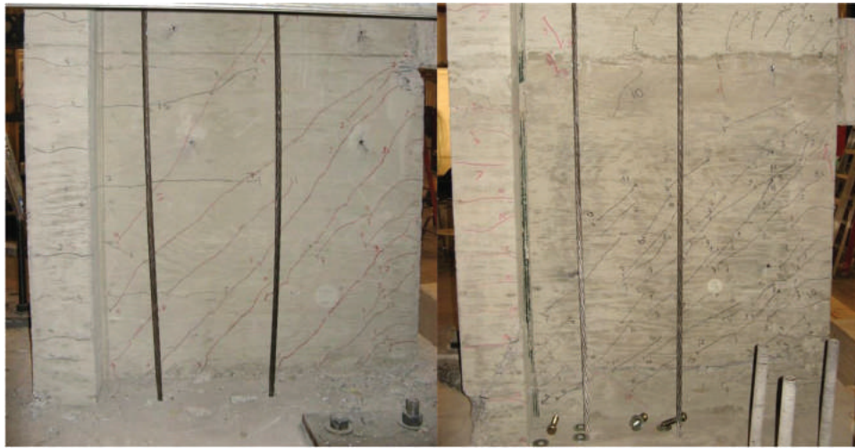
(a) Specimen CW-1 (reinforced concrete)
