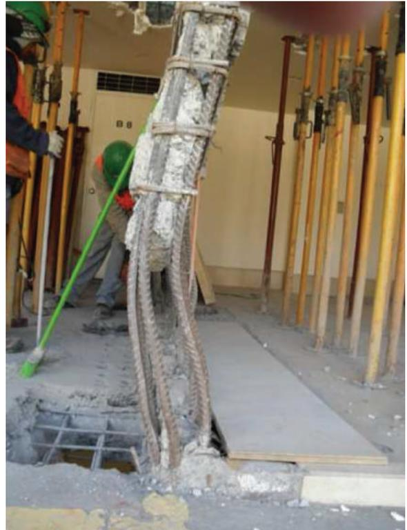
*Fig. 1—Buckled wall at first story of a 15-story building following the 2010 Chile earthquake.*
