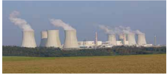
A survey of industry stakeholders indicated a need for inspectors with thorough knowledge of mixture design, concrete constituents, and the performance of concrete after placement
