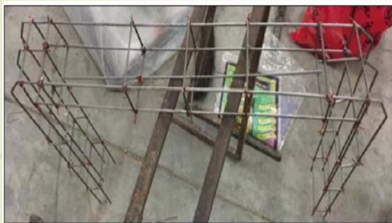
Fig 4 Finished Reinforcement Cage
