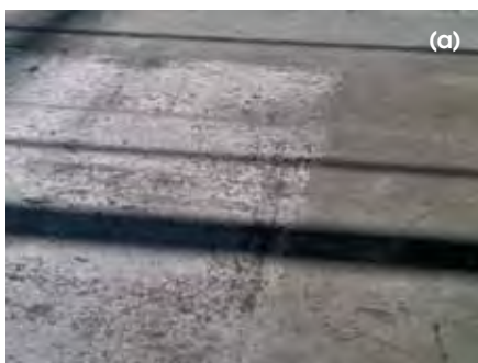
Fig. 1: In many cases, surface moisture problems are associated with the formation of a powder or crystalline residue in areas where tilt-up wall panels were cast: (a) general view of casting area on floor slab; and (b) close-up of crystals
