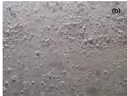
Fig. 1: In many cases, surface moisture problems are associated with the formation of a powder or crystalline residue in areas where tilt-up wall panels were cast: (a) general view of casting area on floor slab; and (b) close-up of crystals
