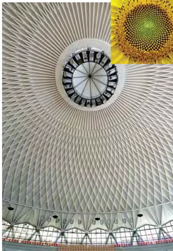
Fig. 9: The small Sports Palace in Rome, Italy, 1957, P.L. Nervi with Antonio Vitellozzi. The elegant pattern of the concrete ribs seems to be inspired by the geometrical network of a sunflower core
