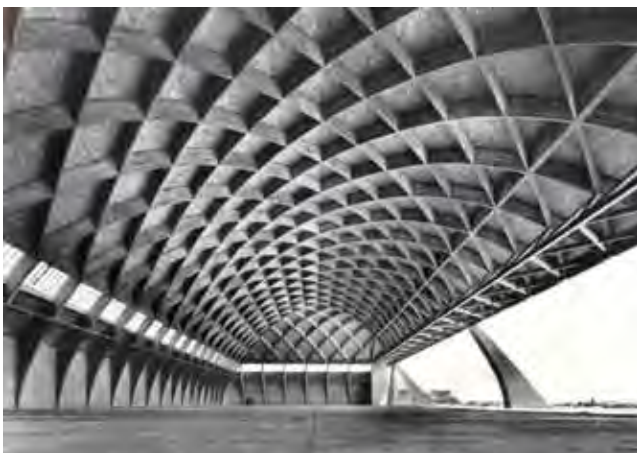
Fig. 3: Hangar at Orvieto, 1935
