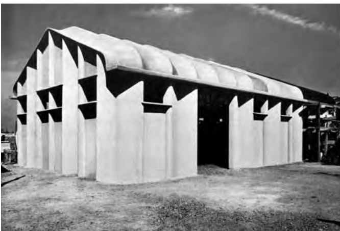
Fig. 6: Nervi reintroduced the use of ferrocement: (left) experimental warehouse in ferrocement, La Magliana, Rome, Italy, 1945; and (right) Pier Luigi Nervi in front of one of his ferrocement boats
