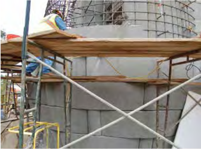
Sixty precast segments were installed to form the exterior of each basket feature
