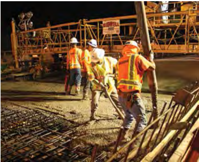
Night placements were necessary to minimize traffic disruption on I-210
