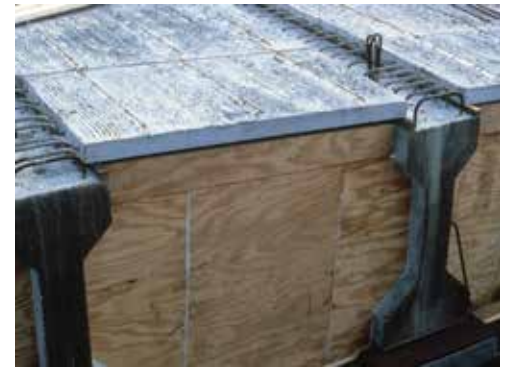
Fig. 15.19: Stay-in-place precast concrete deck forms supported directly on concrete girders
