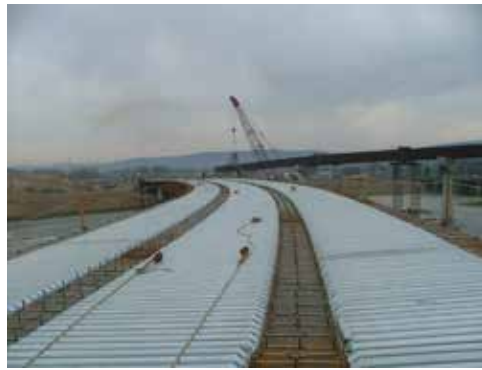
Fig. 15.18: Stay-in-place steel forms attached by self-tapping screws to angle ledgers that have been welded to structural steel bridge girders (Photo courtesy of New York State Department of Transportation©)
